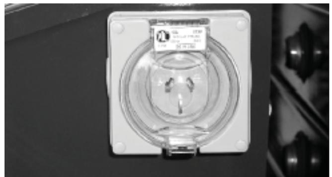
Figure 11.7 - Mains Power Connection For Charger
